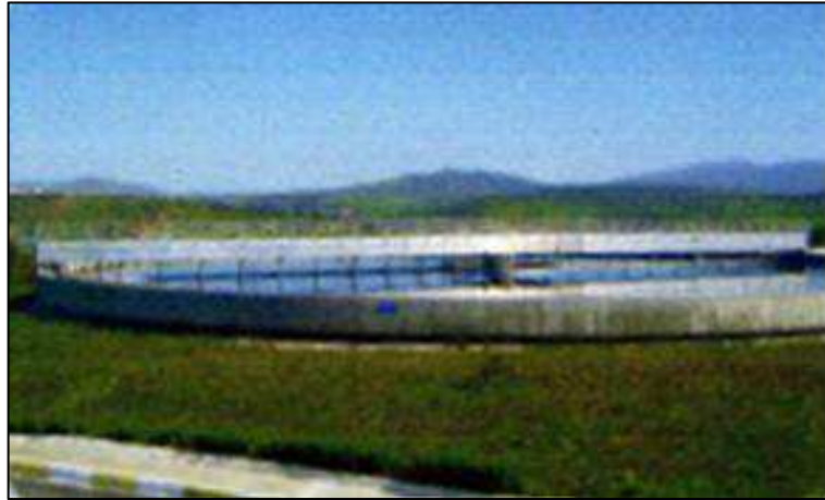
Figure 08: Clarificateur (ONA, 2012).
